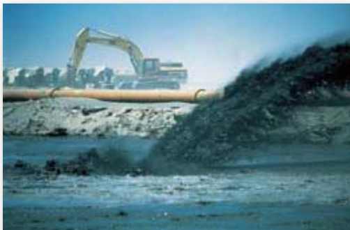
Pipeline end of land reclamation
